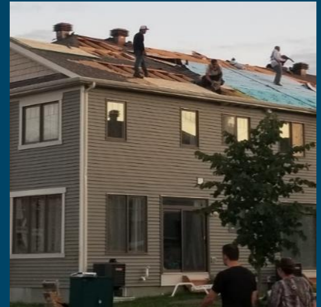
Roof sheathing and shingles blown off during the Barrhaven Tornado on July 13, 2023
